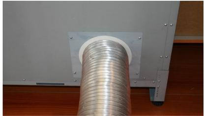
A pipe can be fitted at the side and beneath, measuring 150mm, on both sides and with a choice of two heights (Fig. 1). Extraction at the sides is difficult, and only recommended when the other outlets cannot be used.
