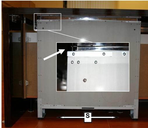
Raise the hood with the legs up until the structure of the hood leans on the kitchen top.
